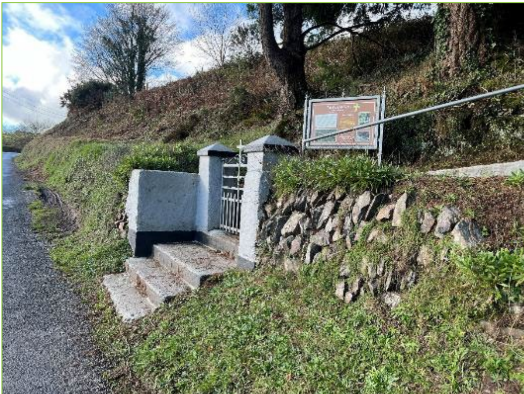
Plate 13.6: View of gateway to footpath leading to mass-rock CO043-009----
